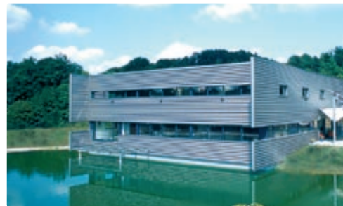
interscience R&D center & manufacturing site Mourjou FRANCE
